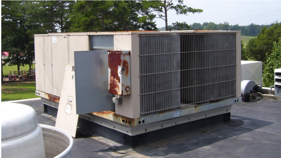
Rooftop HVAC Unit
